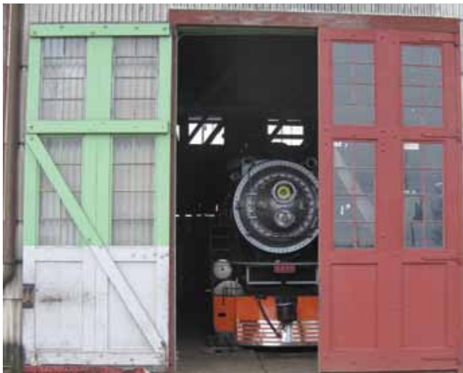
Existing roundhouse doors
